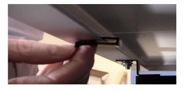
STEP 2: Set the wire mesh screen in place. Make sure the fastener rod comes through the mesh at an upward angle as to keep downward pressure on the screen, pushing it towards the roof.
