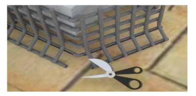
Inner Corner: Secure the first mesh panel in place so it butts up against the solar panel. Cut the bottom fold of the second mesh panel at a 45-degree angle so it does not interfere with the bottom bend of the first panel. Lock in place with Solar Panel Clips. Use corner ties to secure the two mesh panels together.
