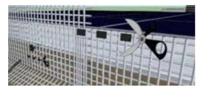
Outer Corner: Cut upwards from the bottom until the bend point. Bend the piece around the corner. Use the supplied stainless steel corner ties to joint the corners.
