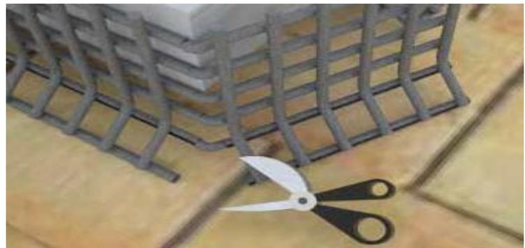
Inner Corner: Secure the first mesh panel in place so it butts up against the solar panel. Cut the bottom fold of the second mesh panel at a 45-degree angle so it does not interfere with the bottom bend of the first panel. Lock in place with Solar Panel Clips. Use corner ties to secure the two mesh panels together.
