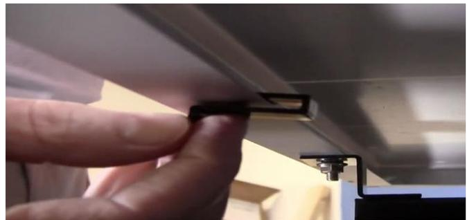
STEP 2: Set the wire mesh screen in place. Make sure the fastener rod comes through the mesh at an upward angle as to keep downward pressure on the screen, pushing it towards the roof.
