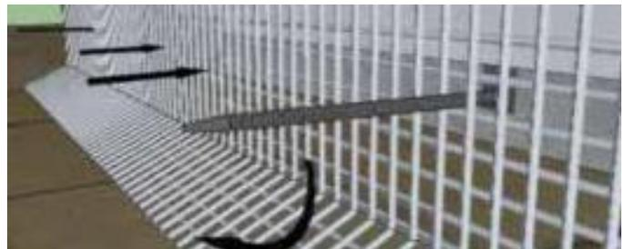
STEP 3: Slide the speed washer and locking nut onto the shaft of the clip assembly until snug. Make adjustments to the screen as necessary with the locking nut. Include a 3” overlap of the mesh when installing the next section and join the mesh with the stainless steel connecting ties.
